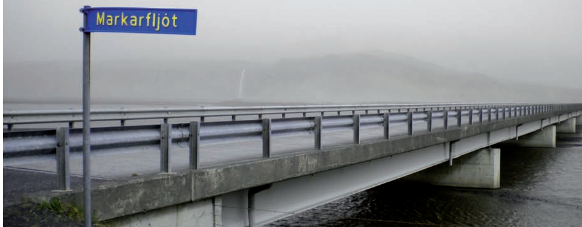
Bridge at Markarfljót on May 25, 2010, looking toward Eyjafjallajökull. Even four weeks after the end of the eruption in Eyjafjallajökull there is still ash in the air, resulting in limited visibility and causing breathing problems for some people
